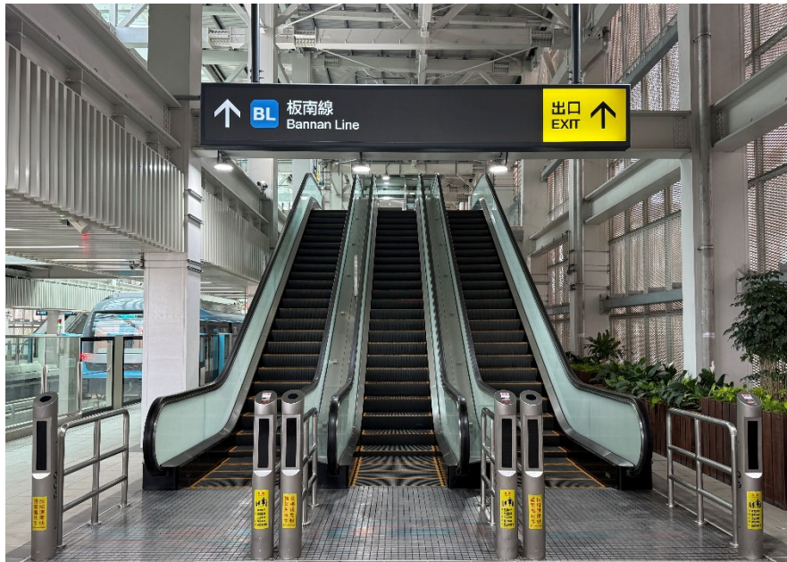
Escalators at Dingpu Station on the New Taipei Metro Sanying Line
